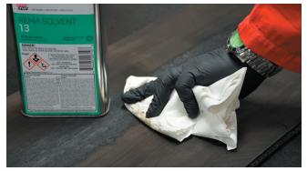
3. Liberally apply cleaning solvent to entire prepared surface, ensuring all contaminants creating during buffing are removed. Allow to air dry until it evaporates off.
