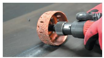
2. Prepare the surface using a buffing tool to achieve a rough profile and remove any lose material. Use the buffing tool to create an angle around the damaged area.
