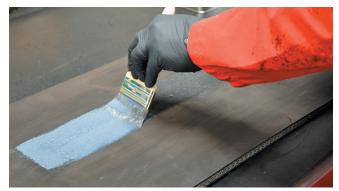
5. Apply first coat of adhesive to prepped surface. Let completely dry for 1 hour.
